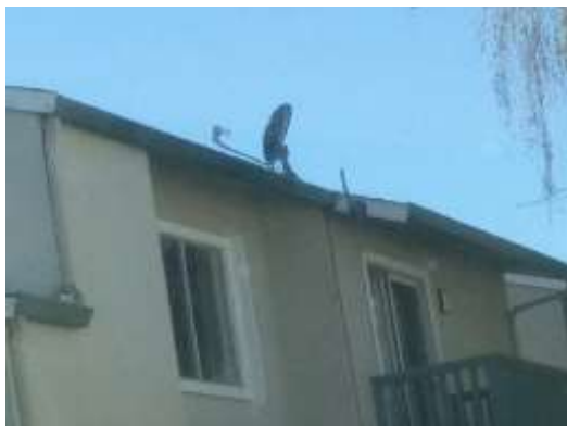
SATELLITE ON ROOF
